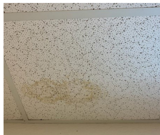
Stained ceiling tiles are a frequent finding, cited under Environment of Care (EC) Standard EC.02.06.01, Element of Performance (EP) 1.
